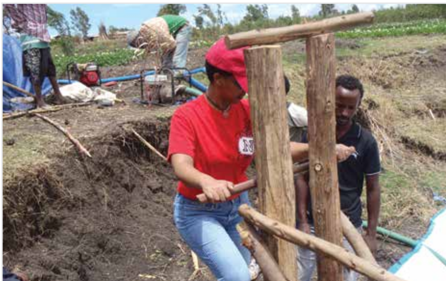
Selected community members were trained on construction and maintenance of the treadle pump (TP) system, including drilling boreholes and installing well casings. Credit: Teshome Regassa
